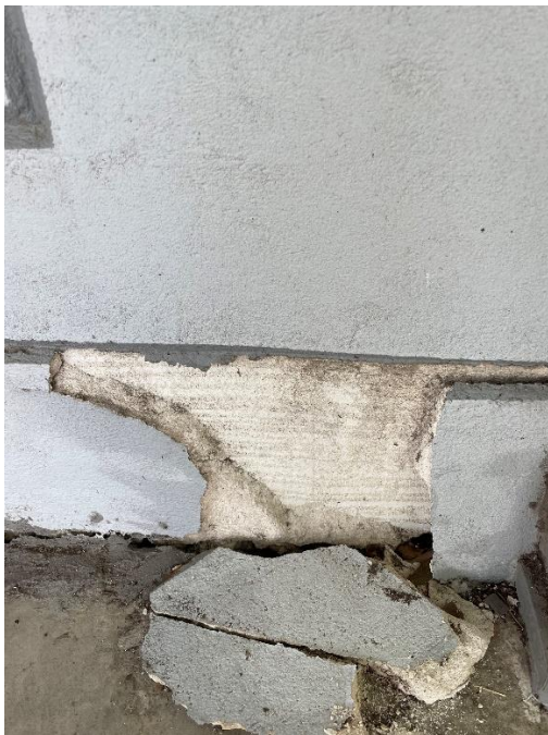
Figure 2. Sampling of the stucco (courtesy of Rubiola Construction).
